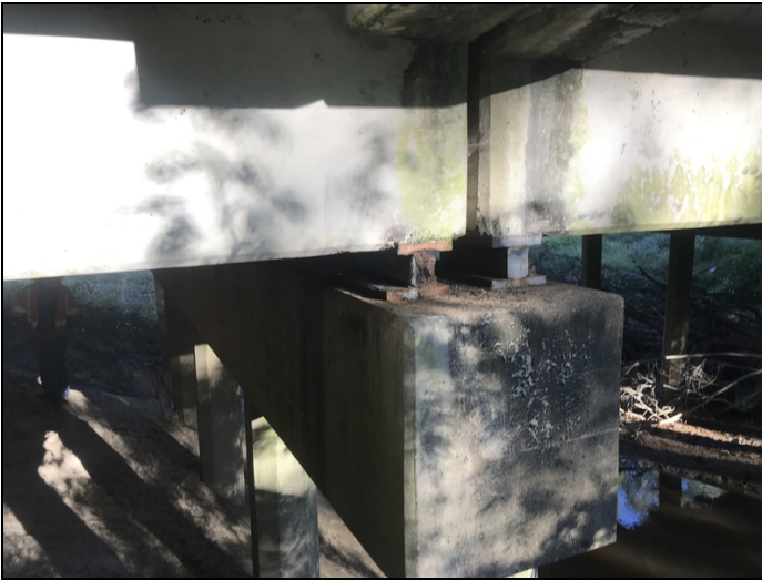
Bent 2 bearing 5 has heavy flaking rust.
