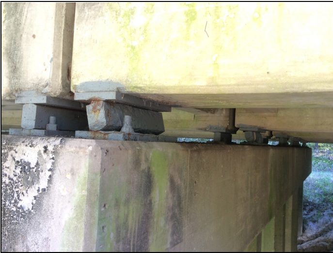
Bent 2 back side bearings (leaning ahead)
