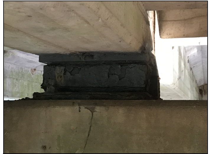
Bent 2 bearing 2 has has heavy flaking corrosion .
