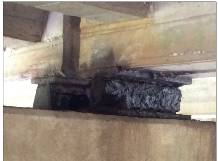
Bent 5 Bearings 3 (corrosion)
