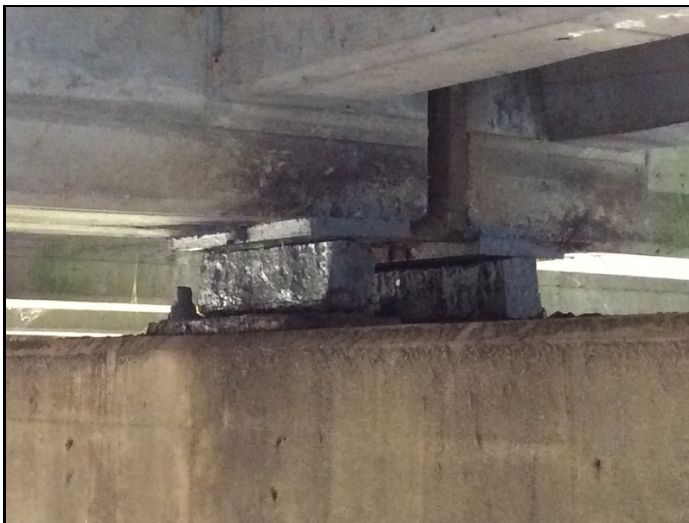
Bent 2 Bearings 4 (corrosion)
