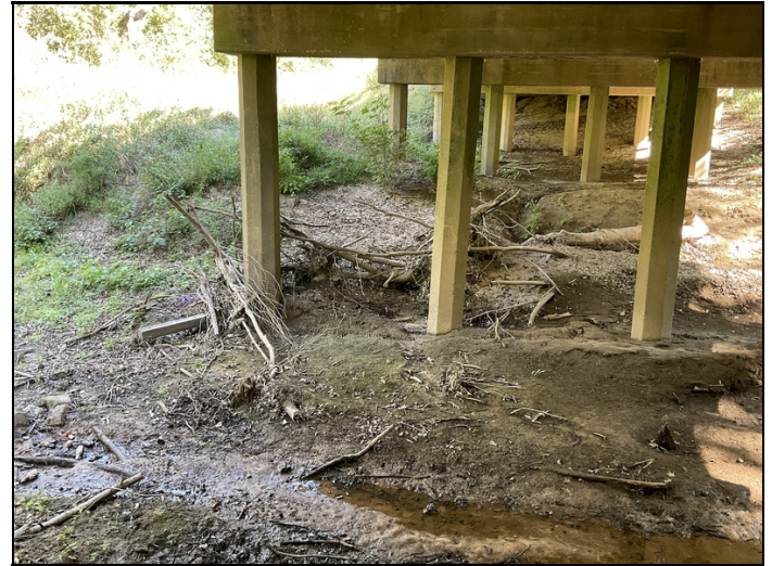
Channel - Bent 3: Debris build-up
