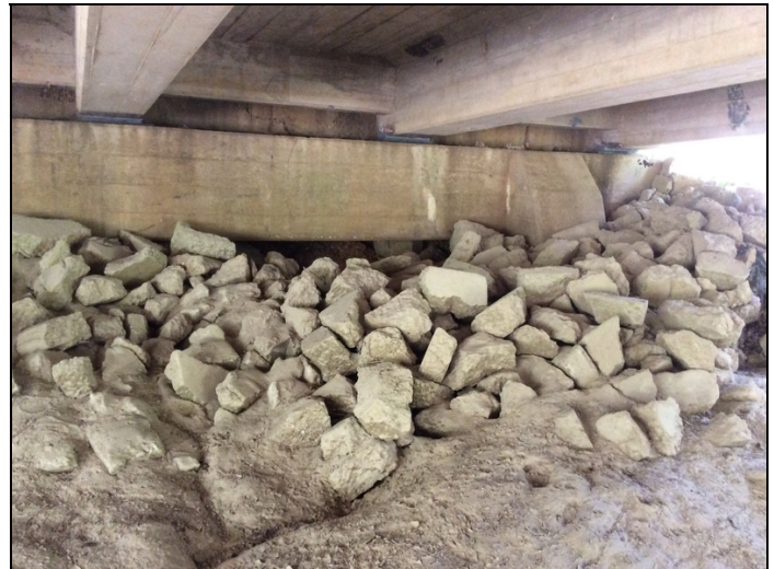
Endslope - Bent 5 right (erosion/settlement)
