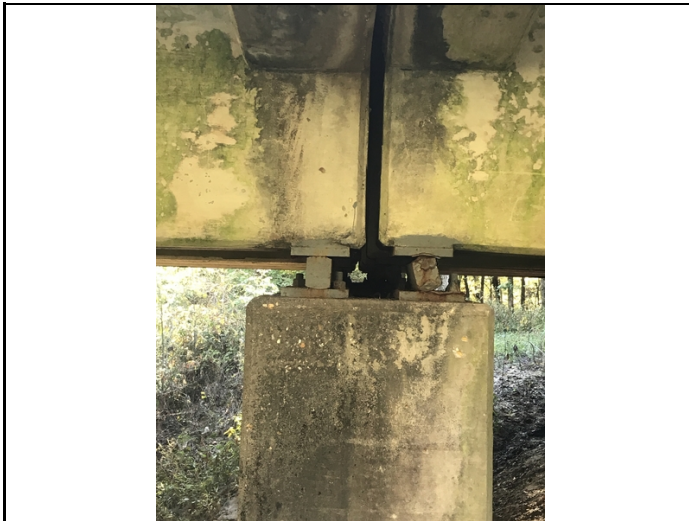
Bent 2 - Bearing 1 left: Corrosion and leaning
