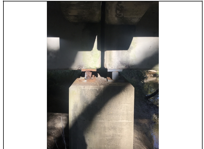
Bent 2 - Bearing 5 right: Corrosion and leaning
