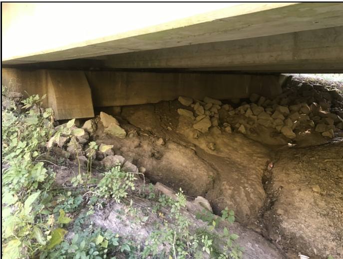
Abutment - Bent 5 : Erosion
