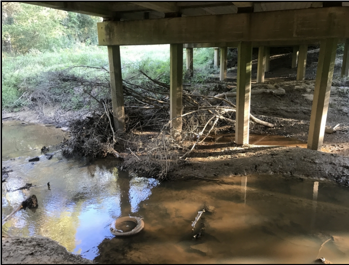
Tree and debris at bent 3 piles .
