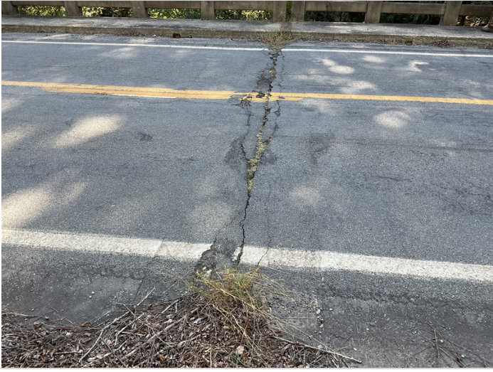
Wearing surface - Bent 2: Spalling
