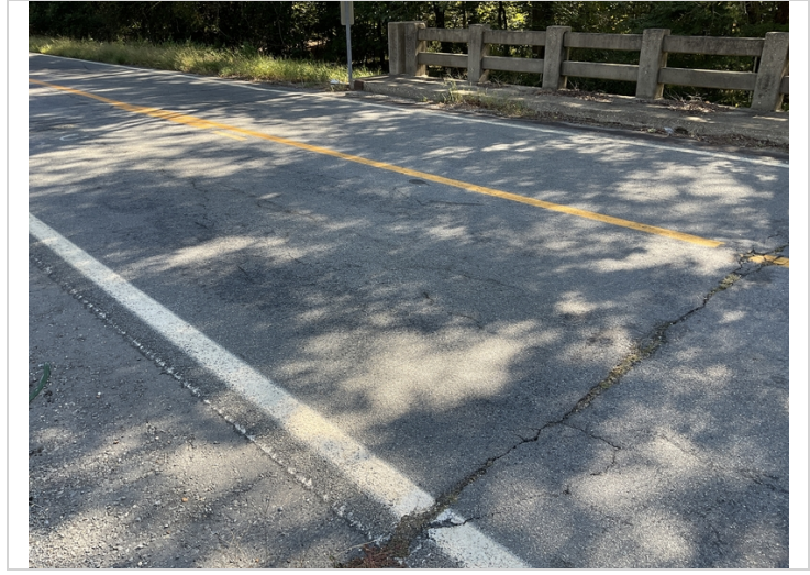
Wearing surface - Span 5: Cracking
