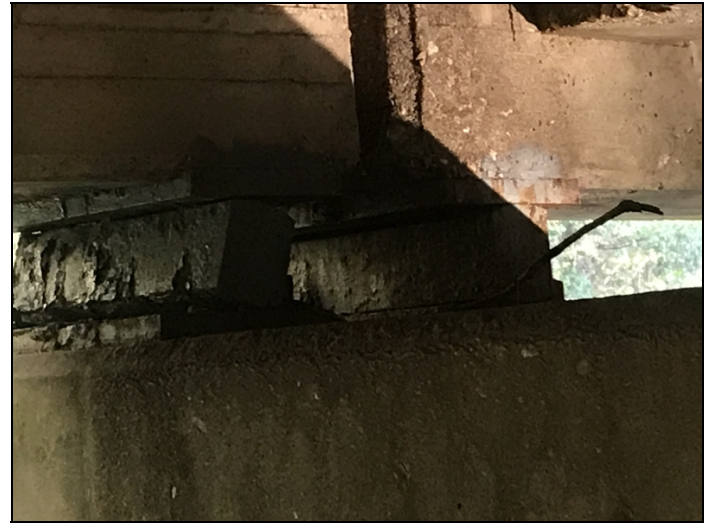
Bent 2 bearing 1 is leaning extremely.
